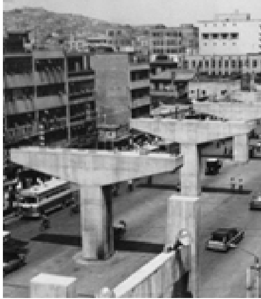
Figure AIII-1 - Example of deck support structure for the BRT. Source: Minhocão Collection - Elevado Costa e Silva - 1970 1 .
