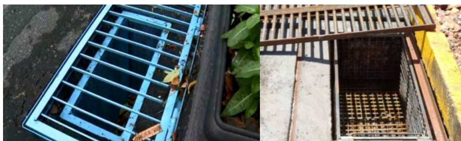
Figure 2: Smart culvert collector models.
