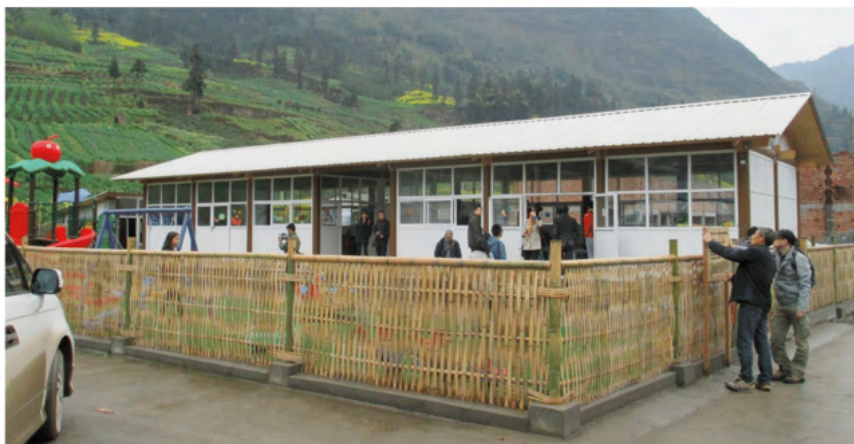
Figura 3 – Escola temporária na China (SHIGERU BAN ARCHITECTS, 2018a, online )
