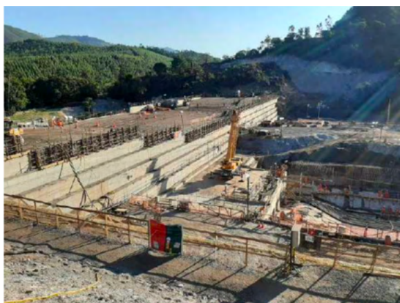
Figure 10. RCC containment dam below Sul Superior.
