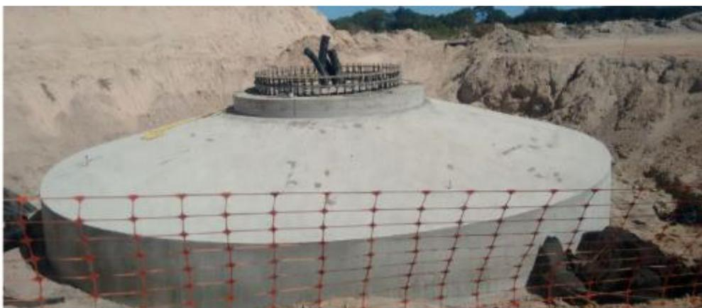
Figura 4 – Sapata concretada (Autores. (2016)).
