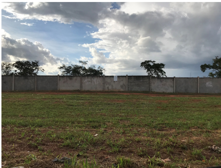
Figura 63 - Wall built by ITV, next to Aldo Borges Leão Avenue, in order to protect its property in Western Sector, Uberlândia -MG, 2019.
