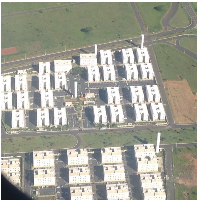
Figure 89 - Aerial image of the United Coast Condominium owned by MRV - Uberlândia –MG, 2015.
