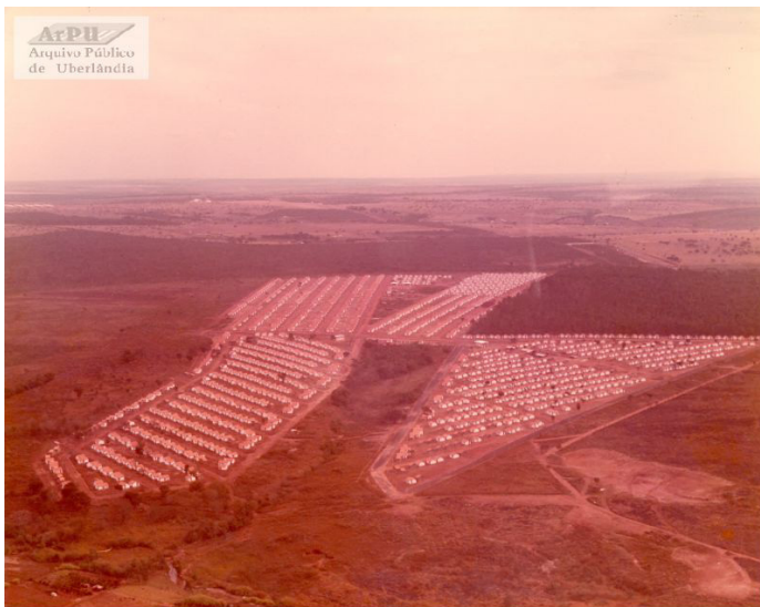
Figure 42 - Luizote de Freitas allotment, late 1970s, Uberlândia-MG. Source: Uberlândia Public Archive (2019).
