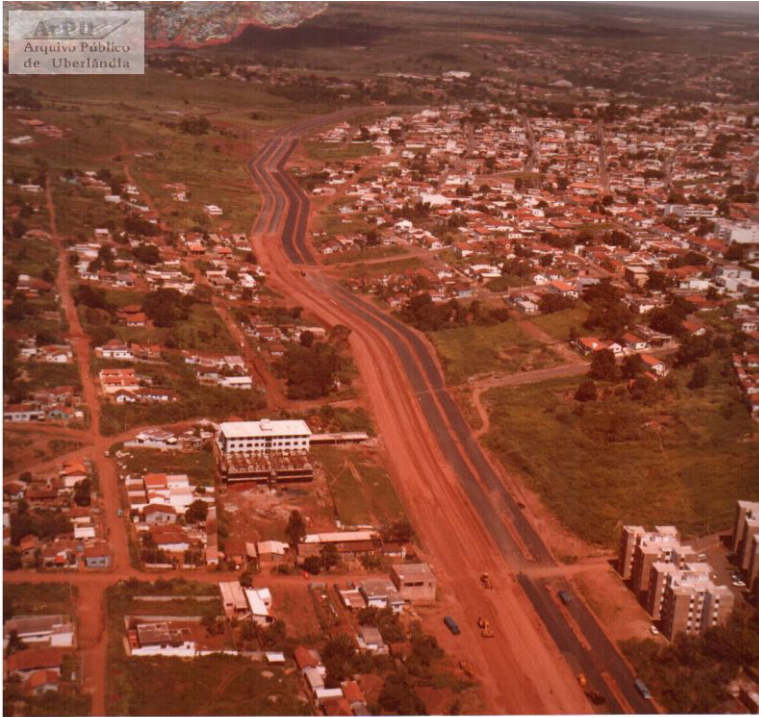
Figure 47 - Canalization work on the São Pedro stream and construction of the Rondon Pacheco Avenue, late 1970s, Uberlândia- MG.
