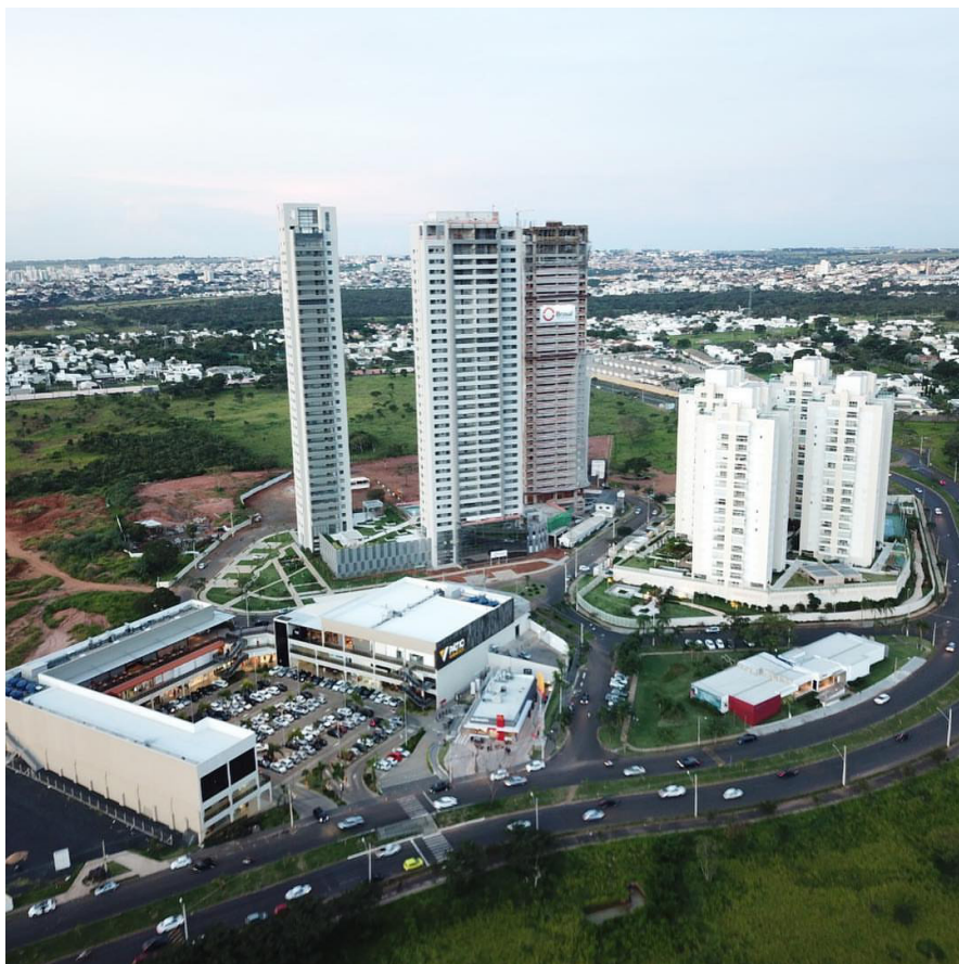
Figure 22 - Aerial view of the Acácias Uberlândia Allotment, Southern Sector, Uberlândia-MG. Source: https://deskgram.net/p/2019144431287164829_384450632 , accessed on 2019, May 09.
