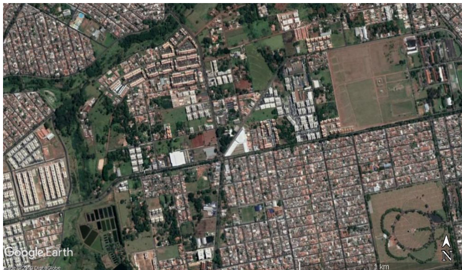
Figure 60 - Aerial image of the Chácaras Tubalina neighborhood, Uberlândia-MG, 2019. Source: Google Earth, accessed on 2019, February 26.
