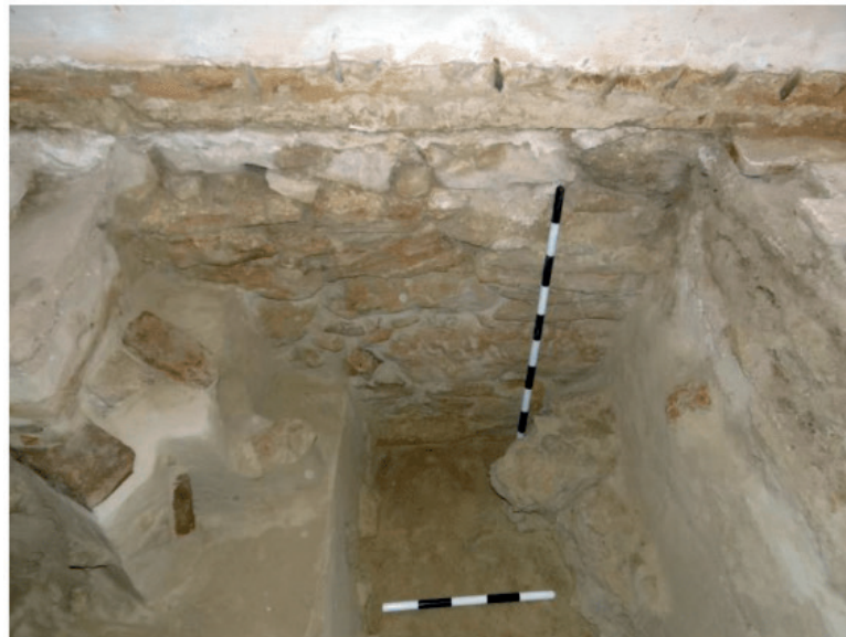
Figure3–Note the foundation with unmortaredjuxtaposed stones.
