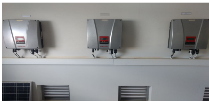
Figura 4 – Inversor INGETEAM modelo Ingecon Sun Lite 3,68TL
