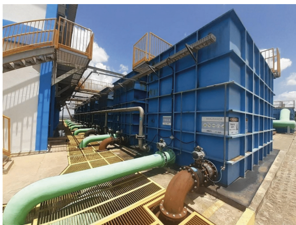
Figure 4 - Arapiraca WTP filters
