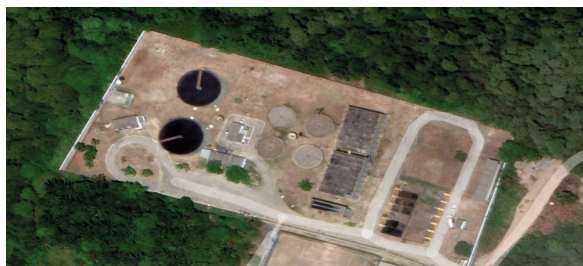
Figure 1 - Dancing Days WWTP (top view).
