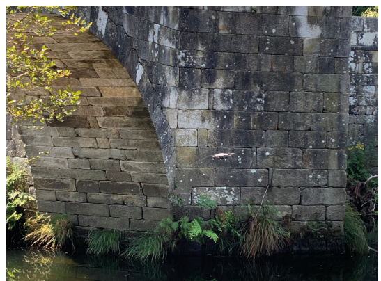
Figure 7 - Multi-rotor drone used in the inspection of the Bandomil Bridge, approaching the upstream elevation of the bridge for inspection of various constituent elements (photo by the author).
