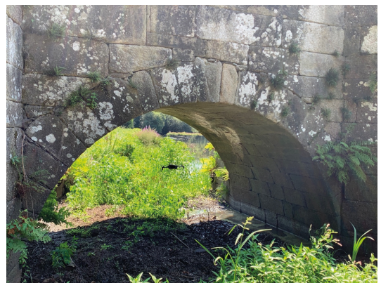
Figure 6 - Multi-rotor drone used in the inspection of the Bandomil Bridge, entering the interior of the minor arch vault for inspection from the upstream side of the bridge (photo by the author).
