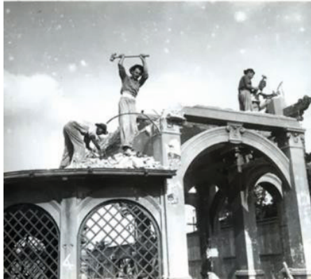
Figure 2: The demolition of the Belvedere.
