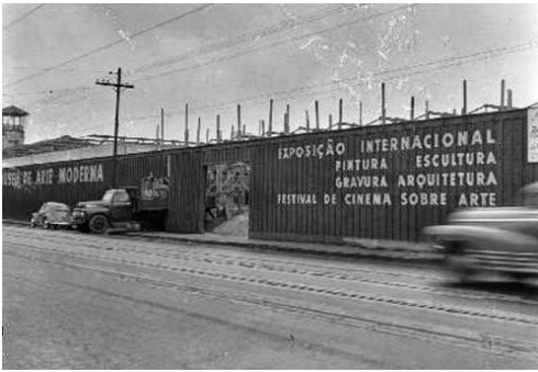
Figure 5: Construction of the pavilion for the first International Art Biennial, 1951.
