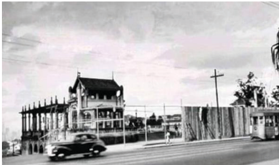
Figure 3: The demolition of the Belvedere.
