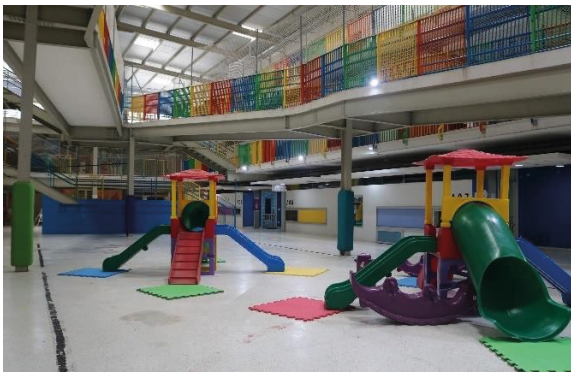
Figure 17: Internal Court yard
