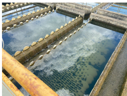
Figure 4: Panorama of the decanter lamellar system
