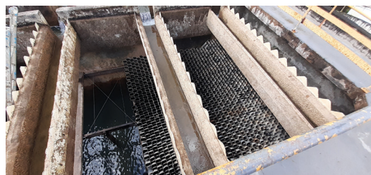
Figure 5: Application of steel cable to support profiles
