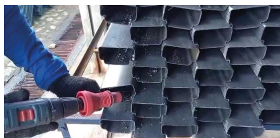
Figure 6: Riveting of lamellar strips
