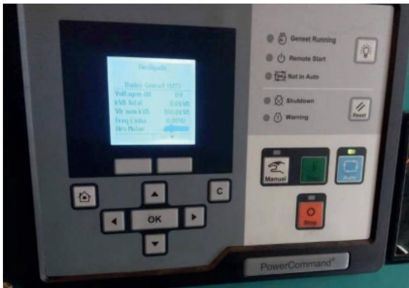
Figura 25 — Controladora PowerCommand
