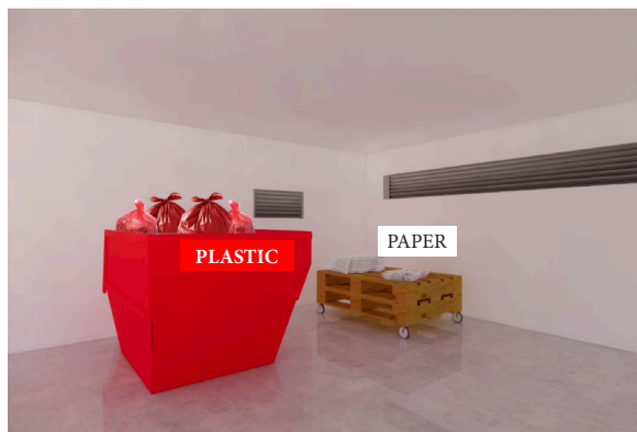
Figure 22: Internal view of the waste storage shelter.
