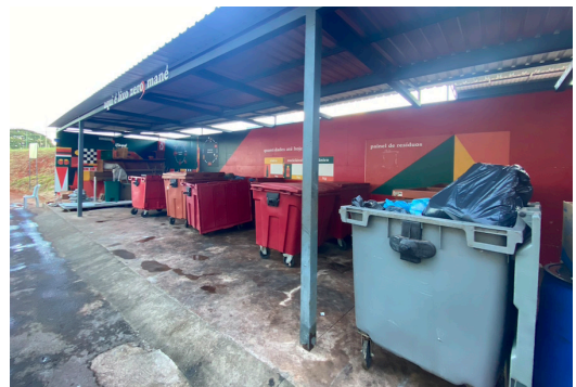
Figure 16: Disposal of waste in containers at the Mané waste shelter.
