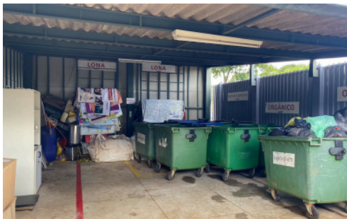
Figure 2: CEUB waste shelter.
