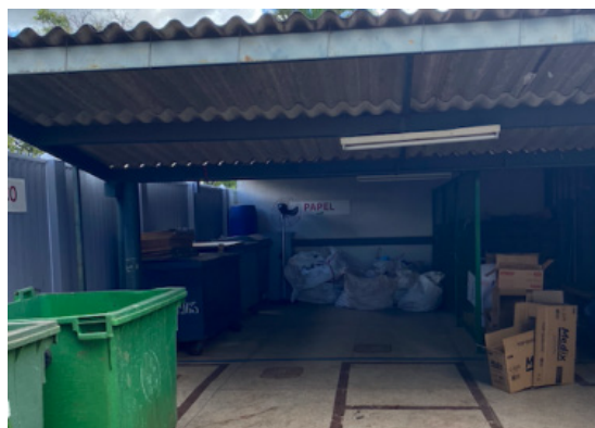
Figure 1: CEUB waste shelter.
