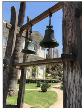
Fig. 3. Temporary support for the bells
