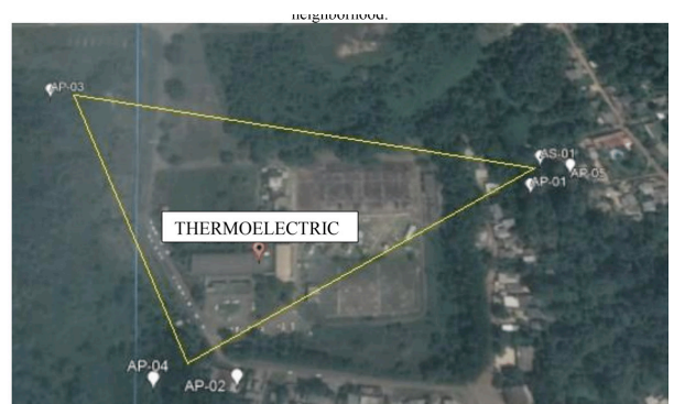
Figure 03. Rio Madeira Thermoelectric Plant in the Nacional neighborhood.
