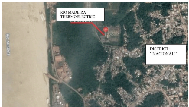
Figure 01. Rio Madeira Thermoelectric Power Plant in the Nacional neighborhood.
