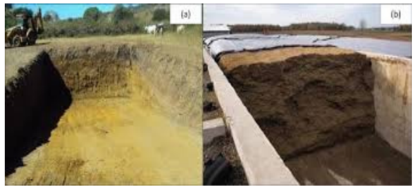
Figure 3. Open half-slope silo.
