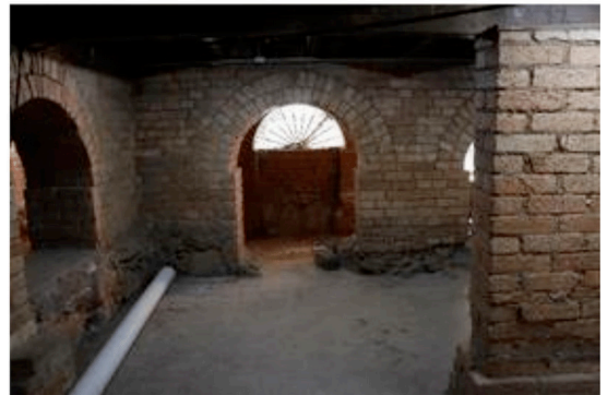
Figure 2: Underground where we see the use of brick in the infrastructure and base of the walls
