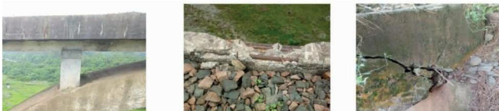
Figure 4 Superstructure pathologies: torsion cracks, steel corrosion, shear crack at Abutment B
