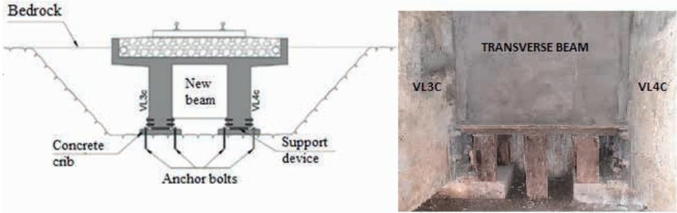
Figure 7 Emergency repair works at abutment B
