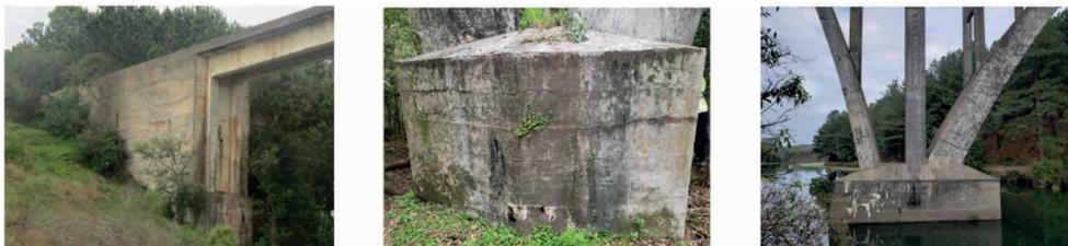
Figure 3 Substructure pathologies: concrete cracking, vegetation, concrete efflorescence
