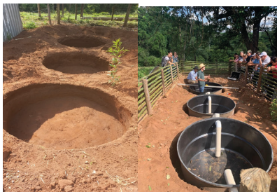
Figure 4 – Installation of the biodigester septic tank.
