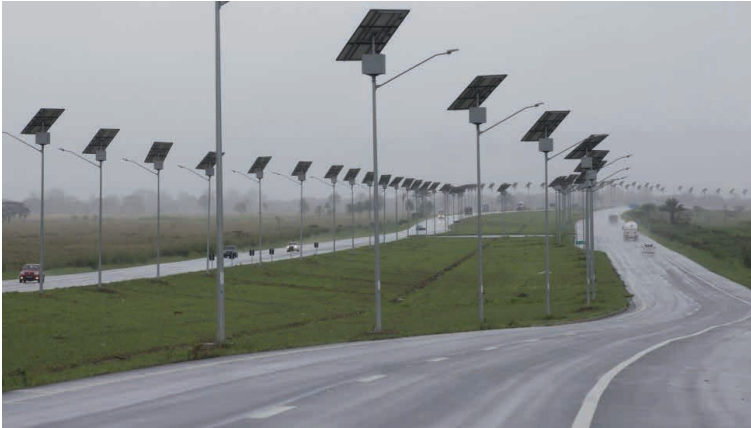
Figure 1 – Poles with solar panels on the Metropolitan Arc of the State of Rio de Janeiro
