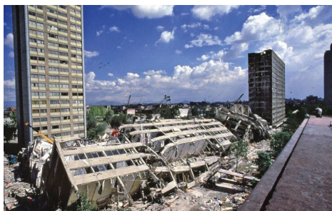
Figure 8: Photo showing the differentiated damage left by an earthquake in the surrounding area depending on the type of construction. The Nuevo León building was completely destroyed and the Veracruz building was not damaged. Different natural frequencies or deficiencies in their construction?
