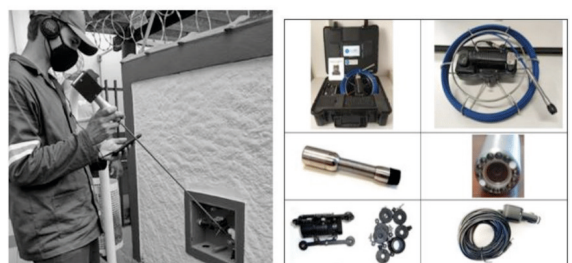
Figure 4 – Search for non-visible leaks – Automated system
