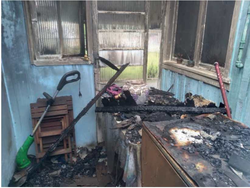
Figure 3. Rear door blocked by furniture
