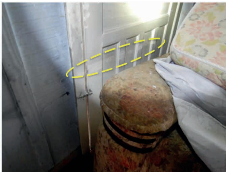
Figure 6. Shadow mark on the door consistent with the height and design of the sofa arm
