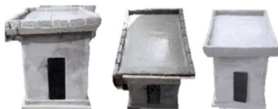
Figure 5. Stages of construction of the prototype roof.
