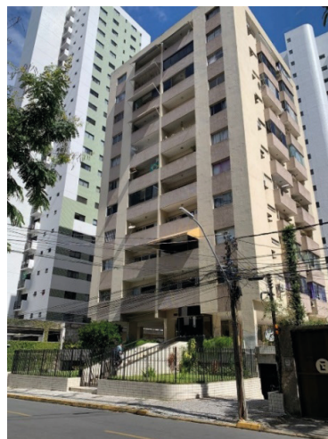
Figure 4 – Front view of the building under study
