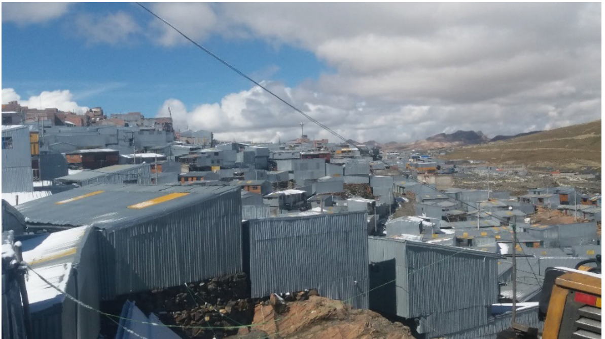
Photo 3. View of houses scattered one on top of the other, built and roofed with calamine, despite the intense cold that the place presents.
