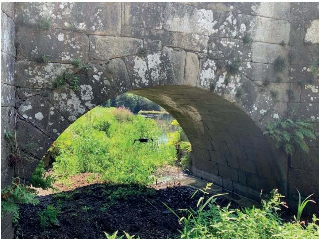
Figure 6: Multi-rotor drone used in the inspection of the Brandomil Bridge, entering the interior of the vault of the minor arch for inspection from the upstream side of the Bridge (photograph by the author).
