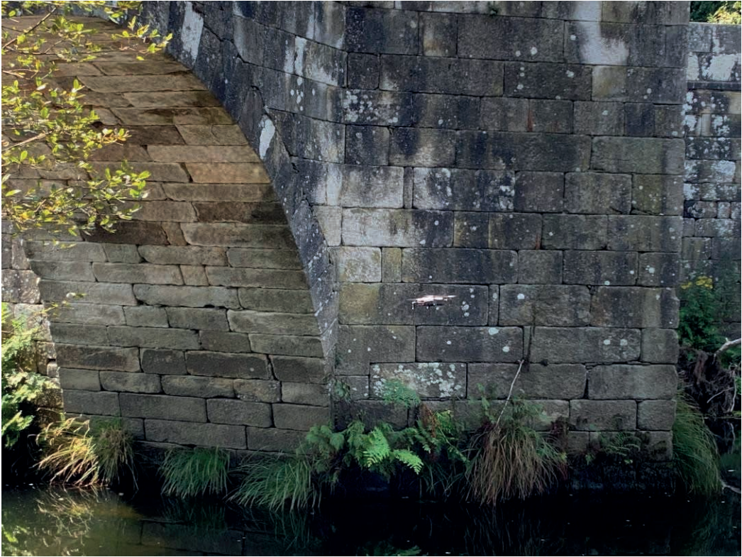
Figure 7: Multi-rotor drone used in the inspection of the Brandomil Bridge, approaching the upstream elevation of the Bridge, for the inspection of various constituent elements (photograph by the author).
