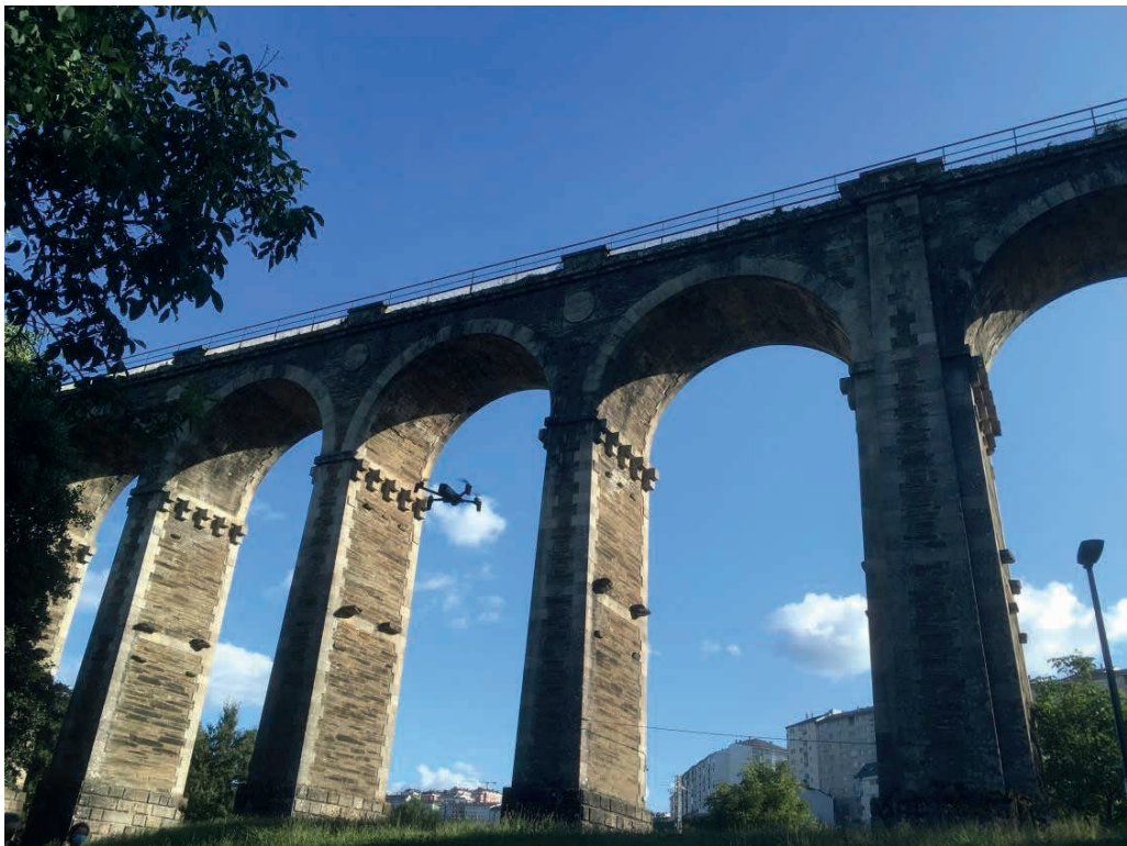
Figure 2: Quadcopter drone approaching for an inspection over the Ponte da Chanca, a railway viaduct located in the city of Lugo that celebrated its 150th anniversary on December 20, 2021 (photograph by the author).
