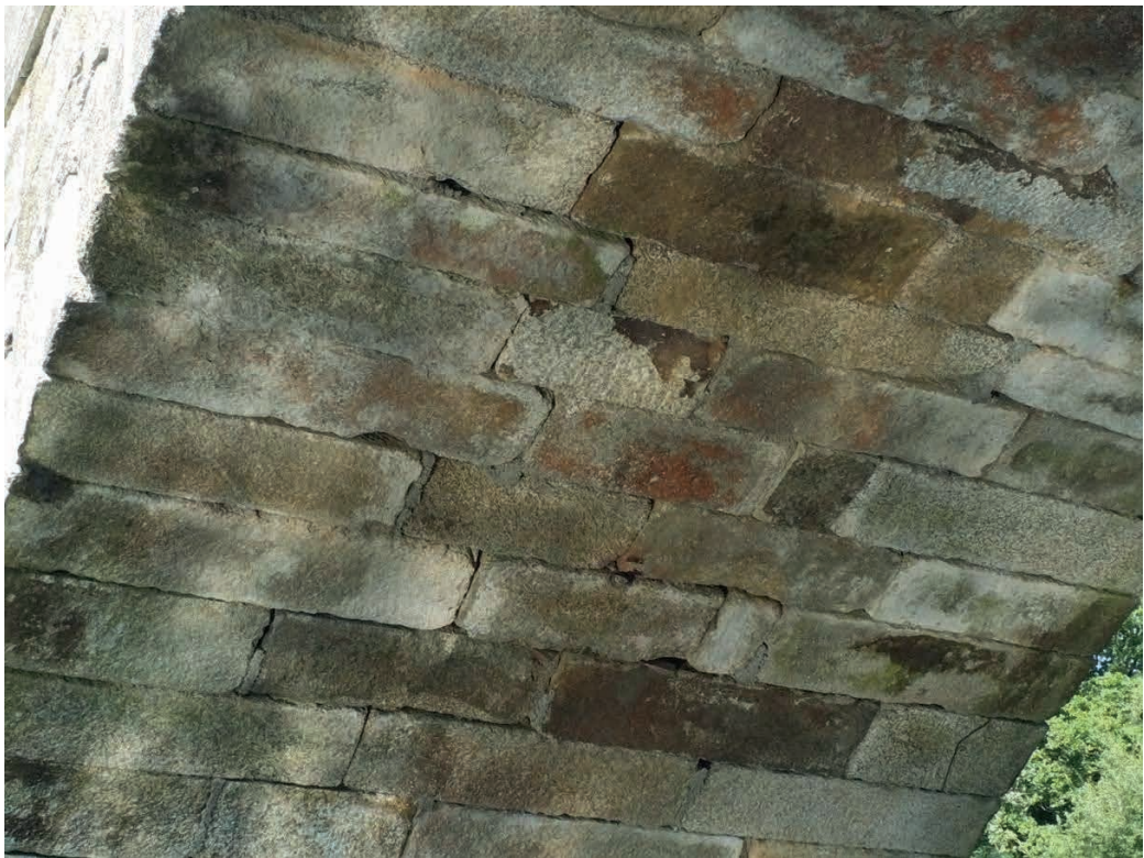
Figure 8: General view of the downstream elevation of the Brandomil Bridge, in an image captured with the multi-rotor drone used in the inspection of this article (photograph by the author).
