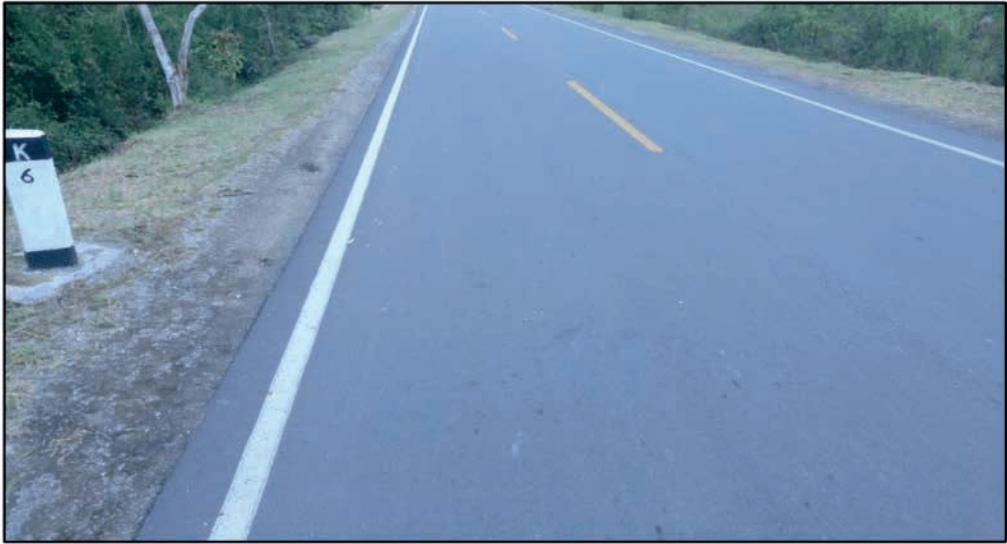
Figura 3 - Pavement surface condition applying nanotechnology
