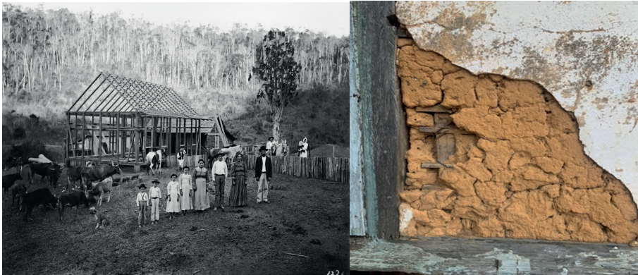
Figure 05- On the left construction of a half-timbered house by immigrants; On the right, hand-made Taipa wall.
