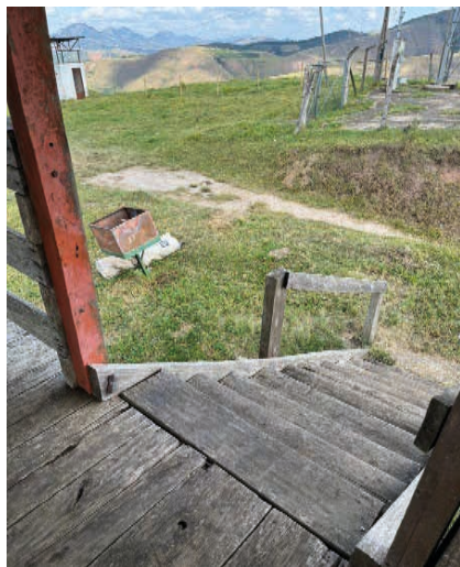
Figure 21 – Railing of the gazebo stairs. SOURCE: Author's collection (2022)
