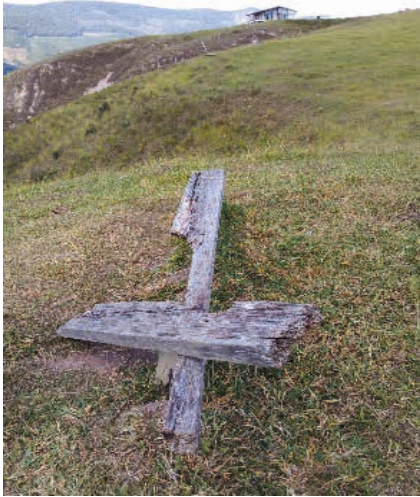
Figure 19 - Broken wooden bench. SOURCE: Author's collection (2022)
