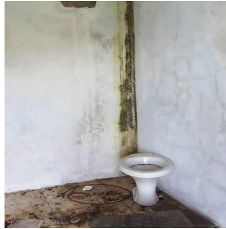
Figure 24 - Condition of the bathroom – Internal photo
