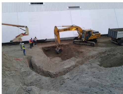
Figure 11 . Beginning of earthworks in August 2016. Source: Personal collection.
