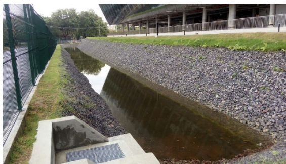
Figure 20 . Retention basin after intense rainy event (November/2017). Source: Image courtesy of the private collection of Phytostore Brasil.
