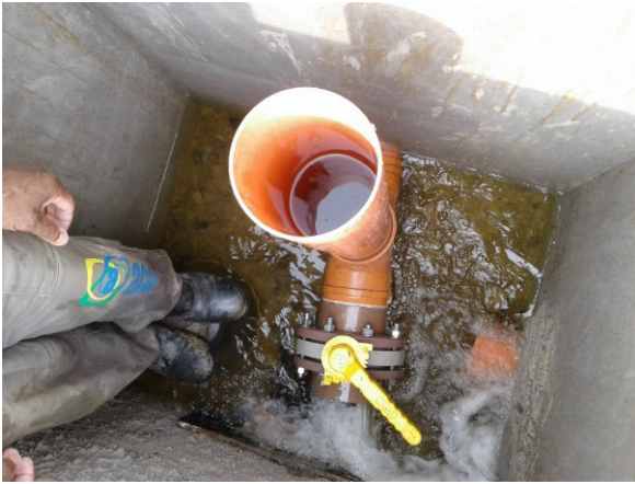
Figure 17 . “Rustic valve”, hydraulic drainage of the filtering garden, March/April 2016. Source: Personal collection.
