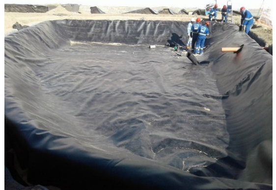
Figure 13 . Installation of the waterproofing blanket in September 2016. Source: Personal collection.
