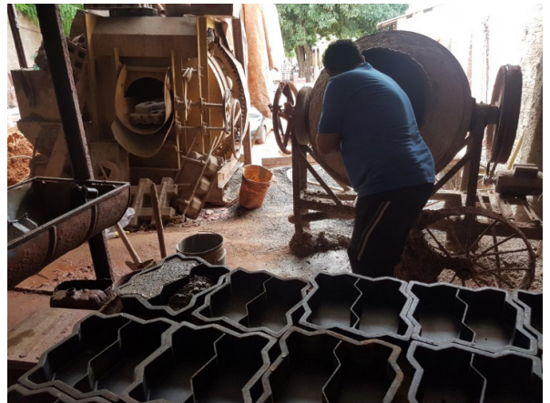
Figure 6. Preparation of interlocking blocks.
