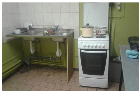
Image 03 – Kitchen on the 2nd floor of the dorm
