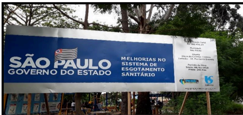
Fig. 1- Work identification plate.
