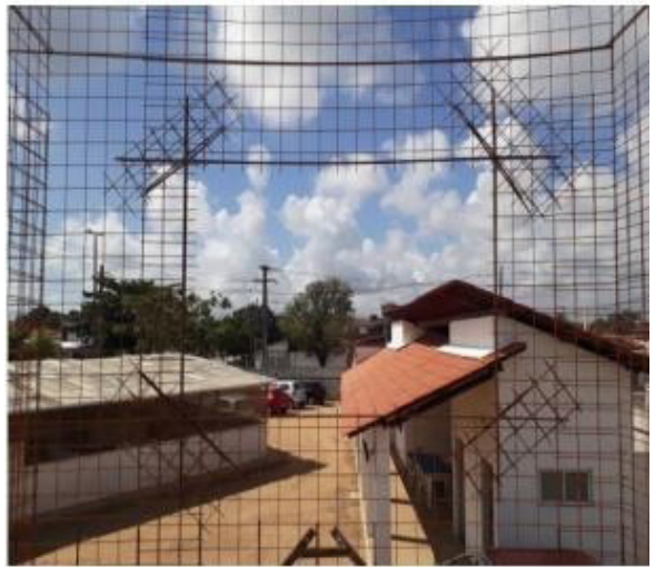
Figure 3. Cutting out the mesh for span of window (Construction Company Archive, 2020).
