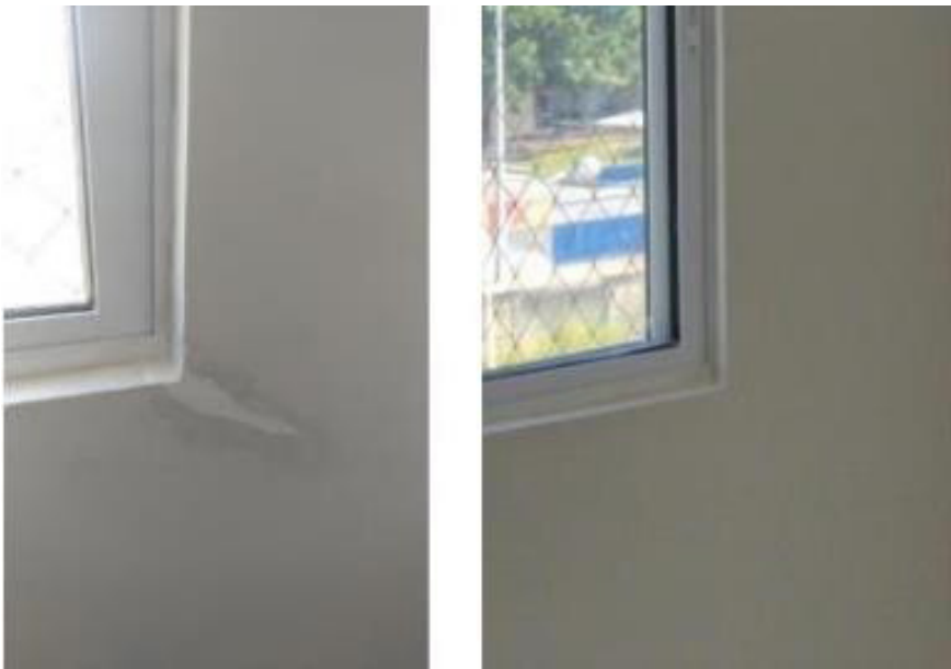
Figure 11. Correcting infiltration in window frames (Construction Company Archive, 2020).
