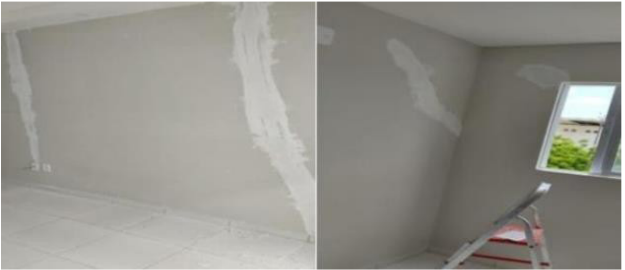
Figure 14. Wall crack repair (Construction Company Archive, 2020).
