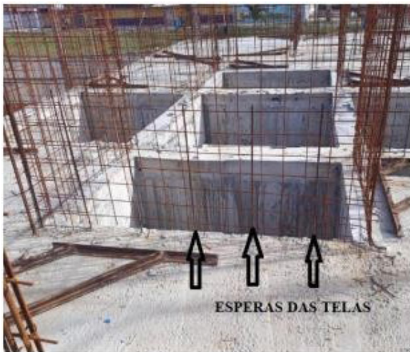
Figure 2. Demarcation of the wall and positioning of the mesh (Construction Company Archive, 2020).
