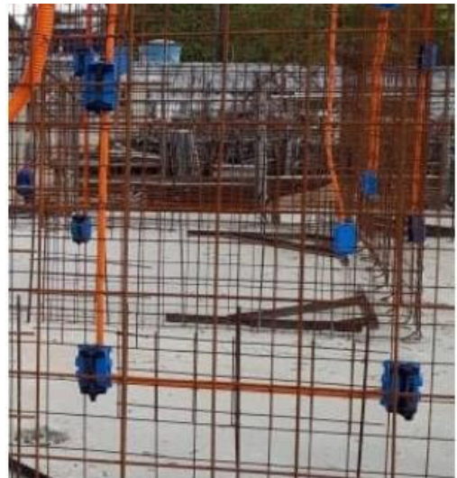
Figure 4. Electrical boxes for walls (Construction Company Archive, 2020).
