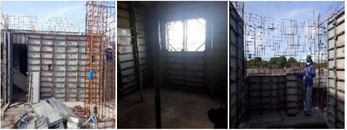
Figure 5. Metallic forms in assembly process (Construction Company Archive, 2020).
