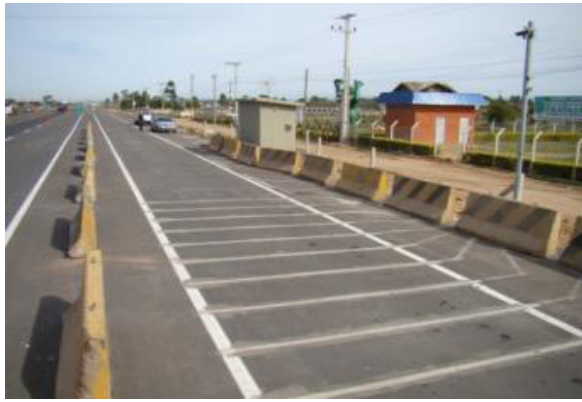
a) After installing the sensors: HS-WIM.
