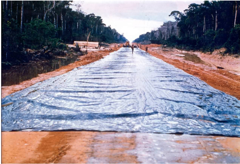
Figure 1 - BR-319 Highway construction
