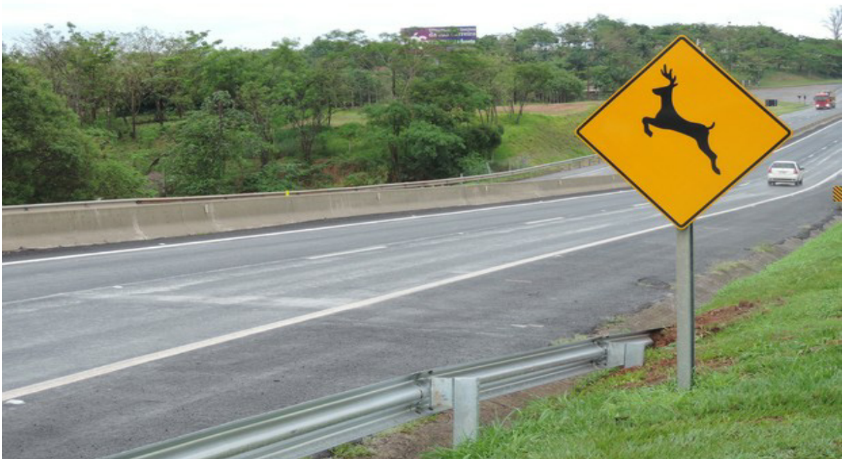
Figure 4 - Concrete barrier divides the lanes of Raposo Tavares Highway (SP-270).
