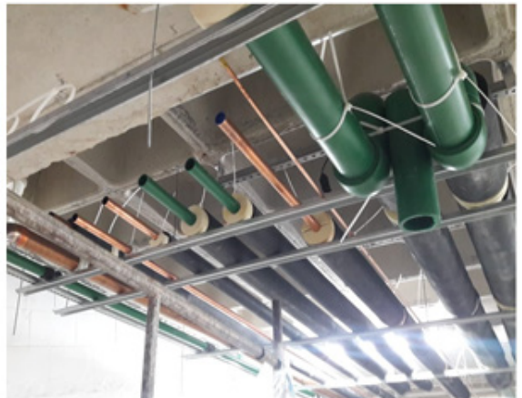
Figure 6. Piping installed underground.
