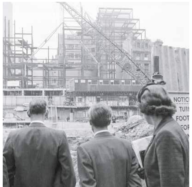
Figure 3: Two men and a woman overlooking a construction site, c.1949–c.1956. Photograph by Nigel Henderson. Black-and-white negative, 5.5 × 5.5 cm. Tate Archive (TGA 201011/3/1/118/5).
