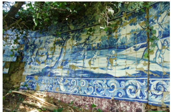
Figure 4 - Panel before the intervention
