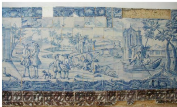
Figure 10 - General appearance of the panels before the intervention.
