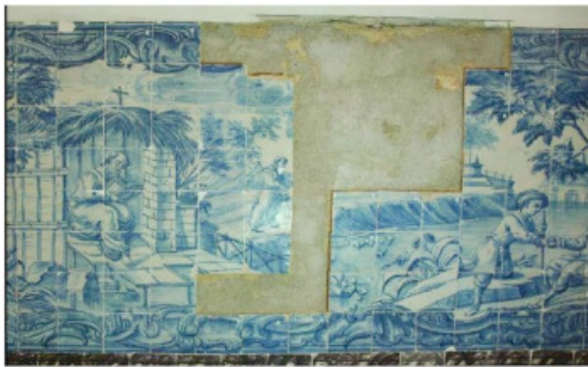
Figure 12 – Wall prepared to receive the new tiles.
