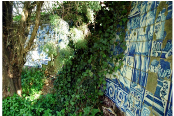
Figure 3 – Panel before the intervention
