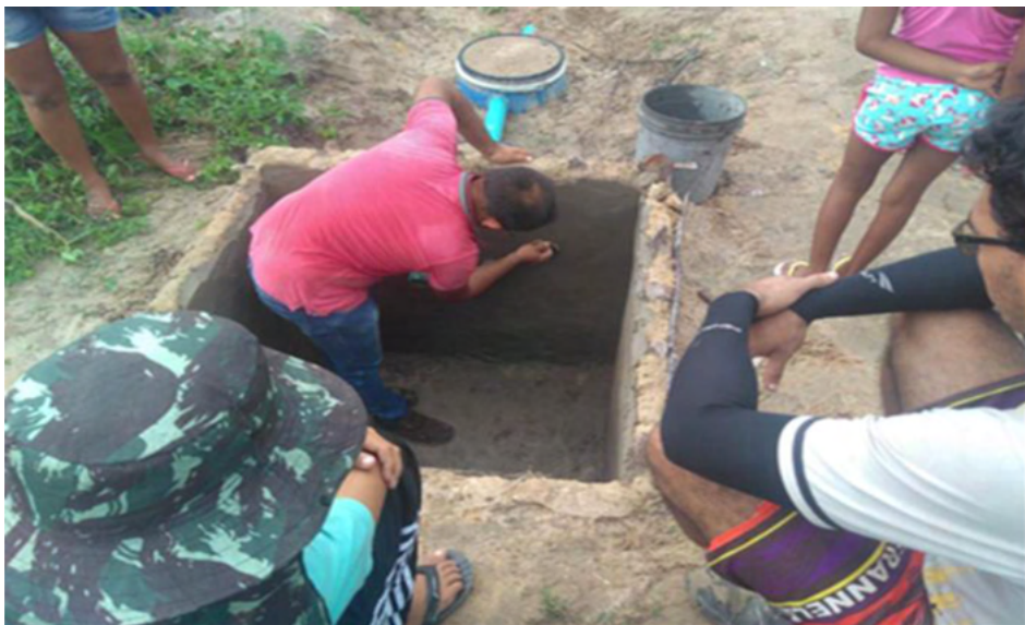
Figure 3. Coating of the evaporator box
