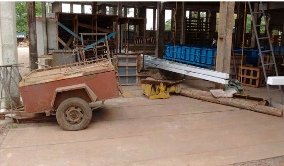
Figure 3 – Cleaning the area next to the Metallurgical.
