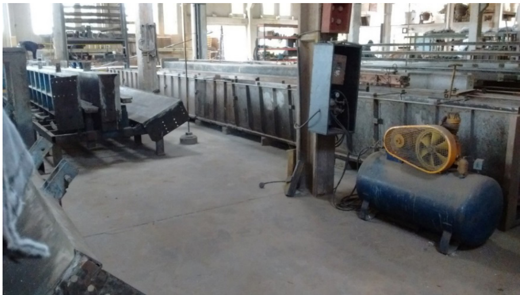
Figure 5 – Cleaning of the sector and removal of the circular saw.
