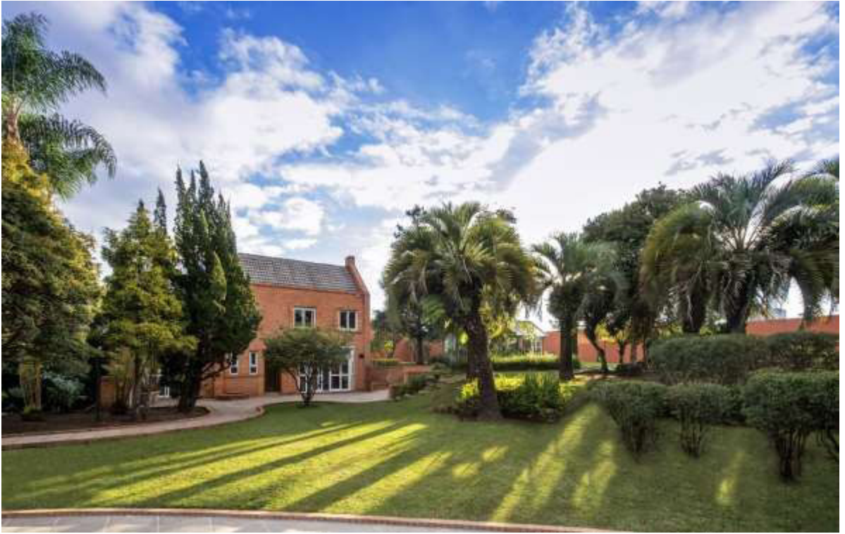
Figure 02. Facade with natural lighting and trees – Hospice Valencis (Curitiba).
