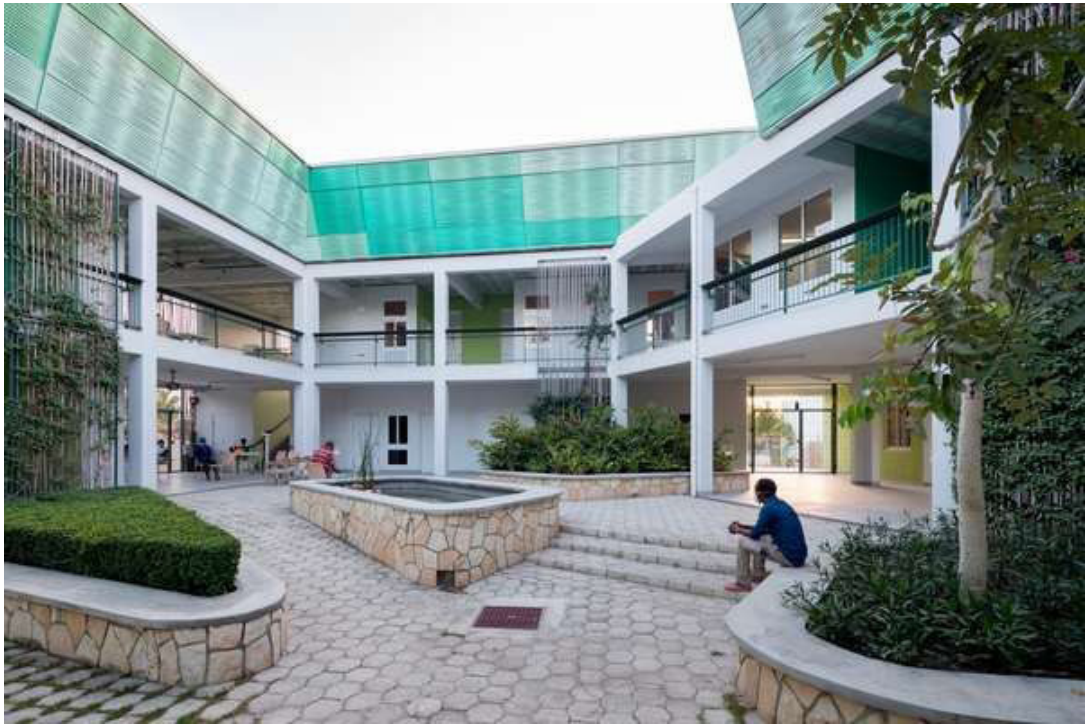
Figure 04. Natural lighting and ventilation – Hospital Gheskio - Haiti.
