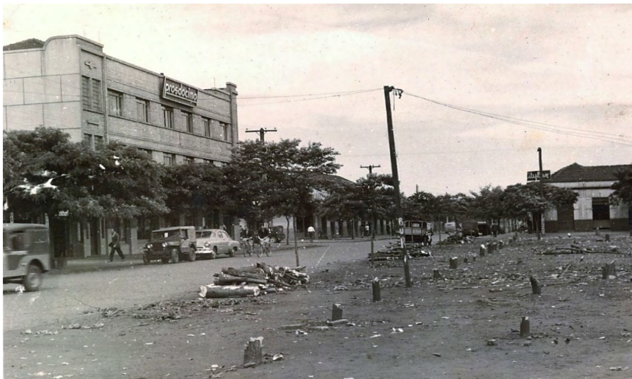
Figure 3: Square after demolition.
