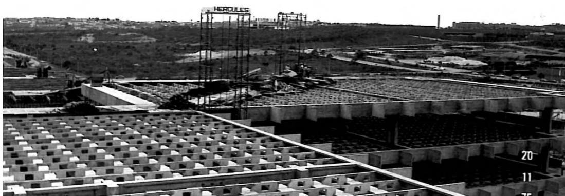
Figure 2. Picture of the construction of the ICB. Source CIT/UFMG, 2019.
