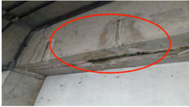
Figure 3.Efflorescence Source: Authors(2018).
