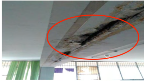
Figure 6. Concrete breakdown
